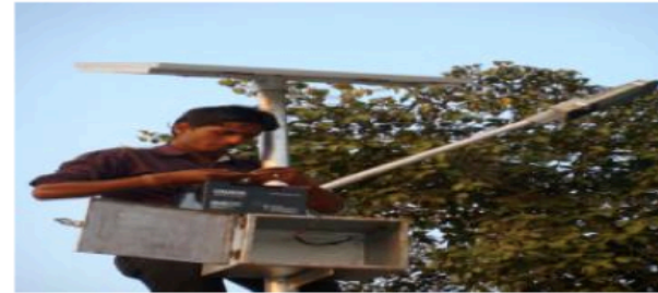
Street lights installed at different locations of Rajasthan and Uttar Pradesh bringing light to the community
