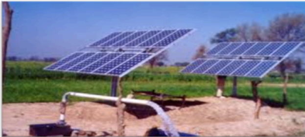
Solar Water pumps installed to help the poor farmers in Rajasthan
