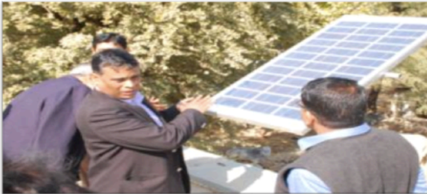
Over 500+ systems installed with support from Baroda Rajasthan Kshetriya Grameen Bank, Rajasthan
