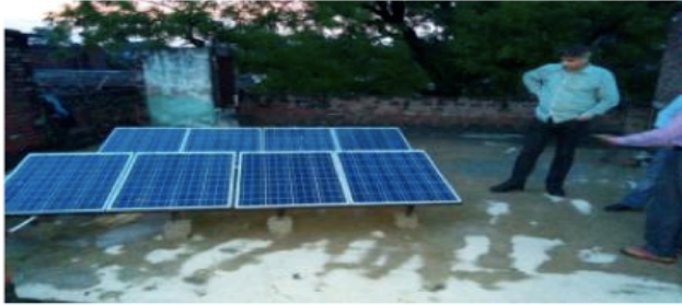
Micro-grids / Mini-grids installed with pre-paid and post paid systems in Uttar Pradesh
