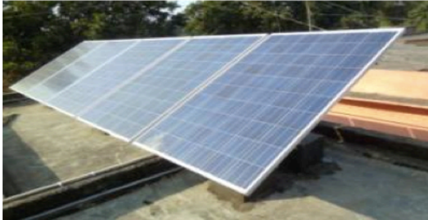
Plant Capacity: 7 KW Location: U.P
