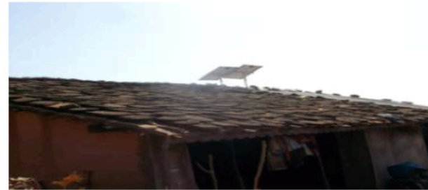
Over 2000 + systems installed in e remote areas of Rajasthan with NGO Mr. Keepi Foundation of Netherlands
